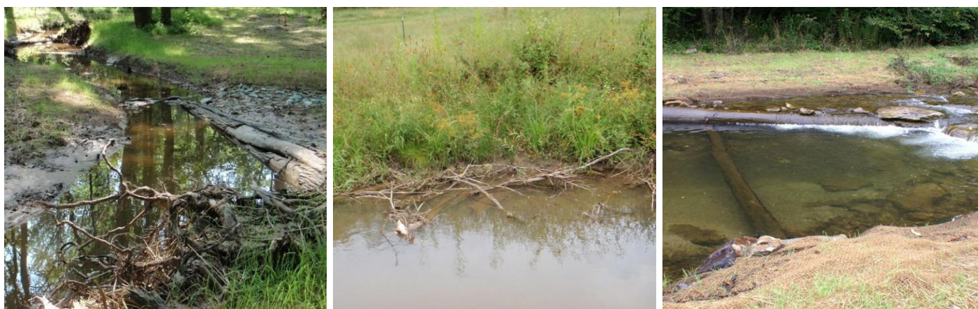
Log vane after a growing season; toe wood structures on stream bank; large woody debris-covered logs. 1
