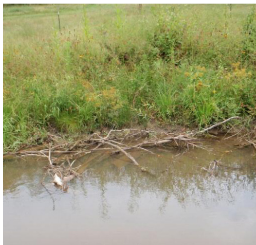
Log vane after a growing season; toe wood structures on stream bank; large woody debris-covered logs. 1
