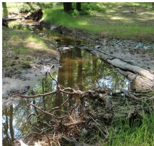
Log vane after a growing season; toe wood structures on stream bank; large woody debris-covered logs. 1
